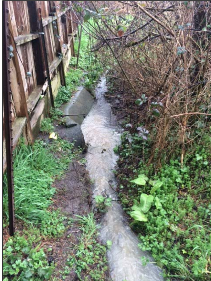
Figure 4.3D Drainage Ditch and 18-inch Concrete Pipe Inlet
