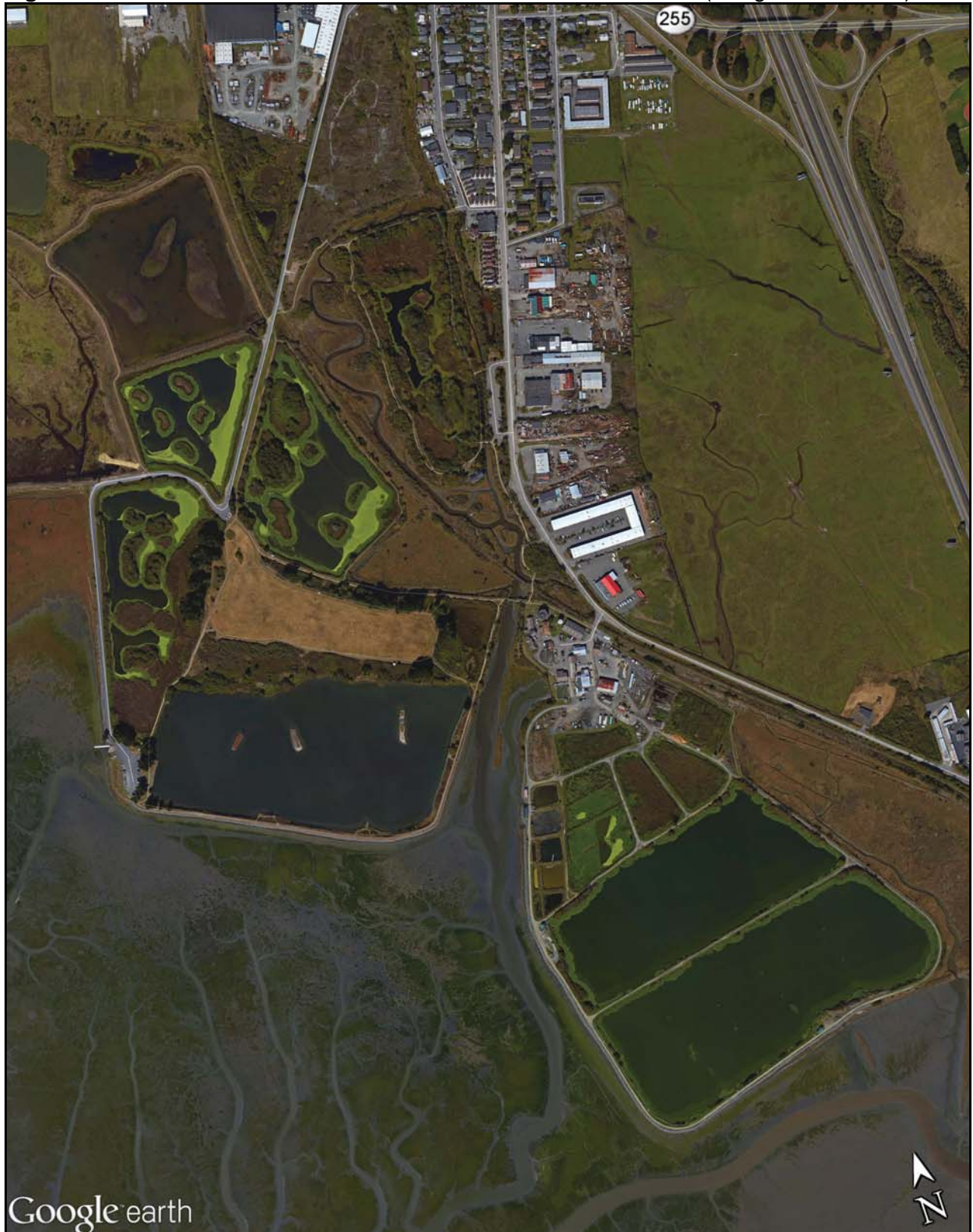
Figure 2.11B Aerial Photo of the Arcata Wastewater Treatment Plant (Google Earth, 2017)
