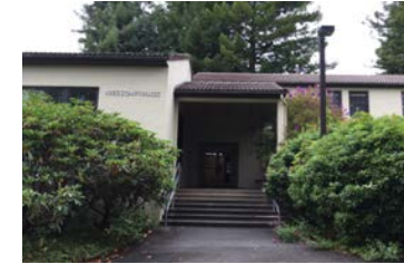
14 Nelson Hall East
