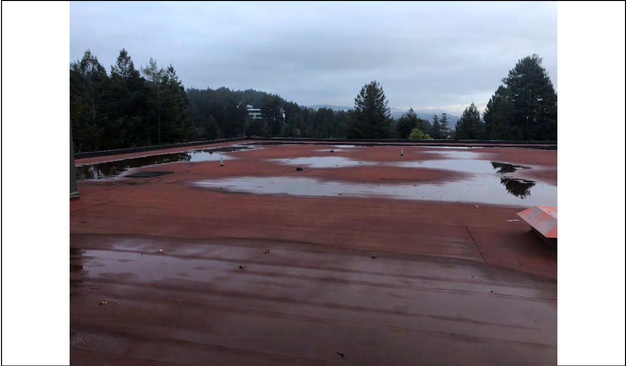
Photograph 2 – Library roof (view looking S)
