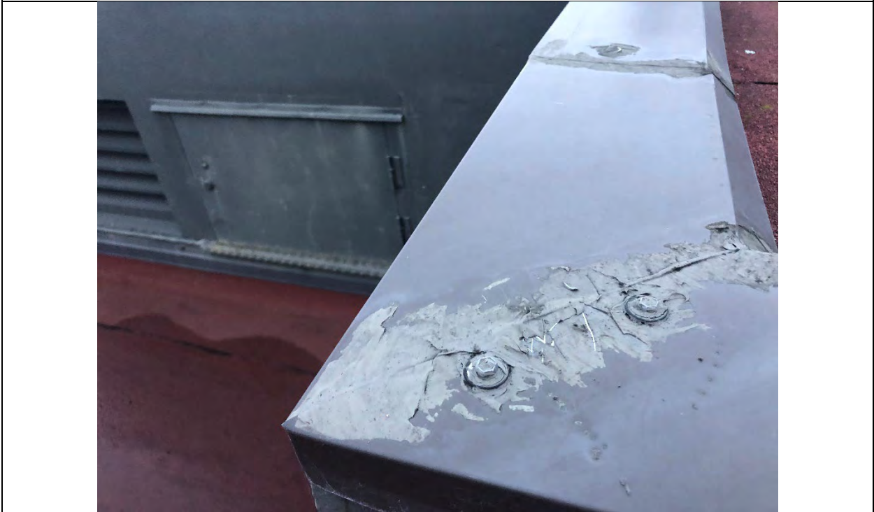
Photograph 6 – Library roof parapet cap flashing seam and fasteners (typical)
