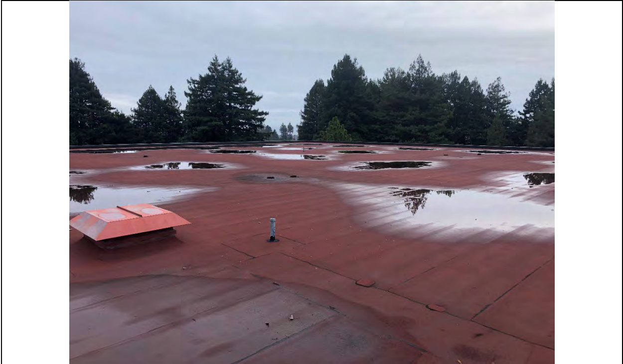
Photograph 1 – Library roof (view looking SW)
