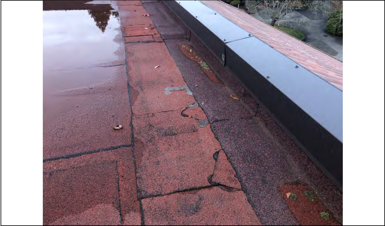
Photograph 5 – Library roof parapet (typical)
