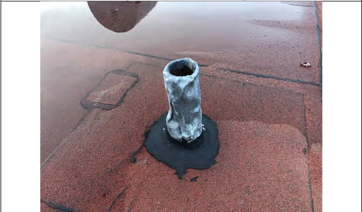
Photograph 4 – Library roof vent (typical) - Metal cladding is presumed to be lead
