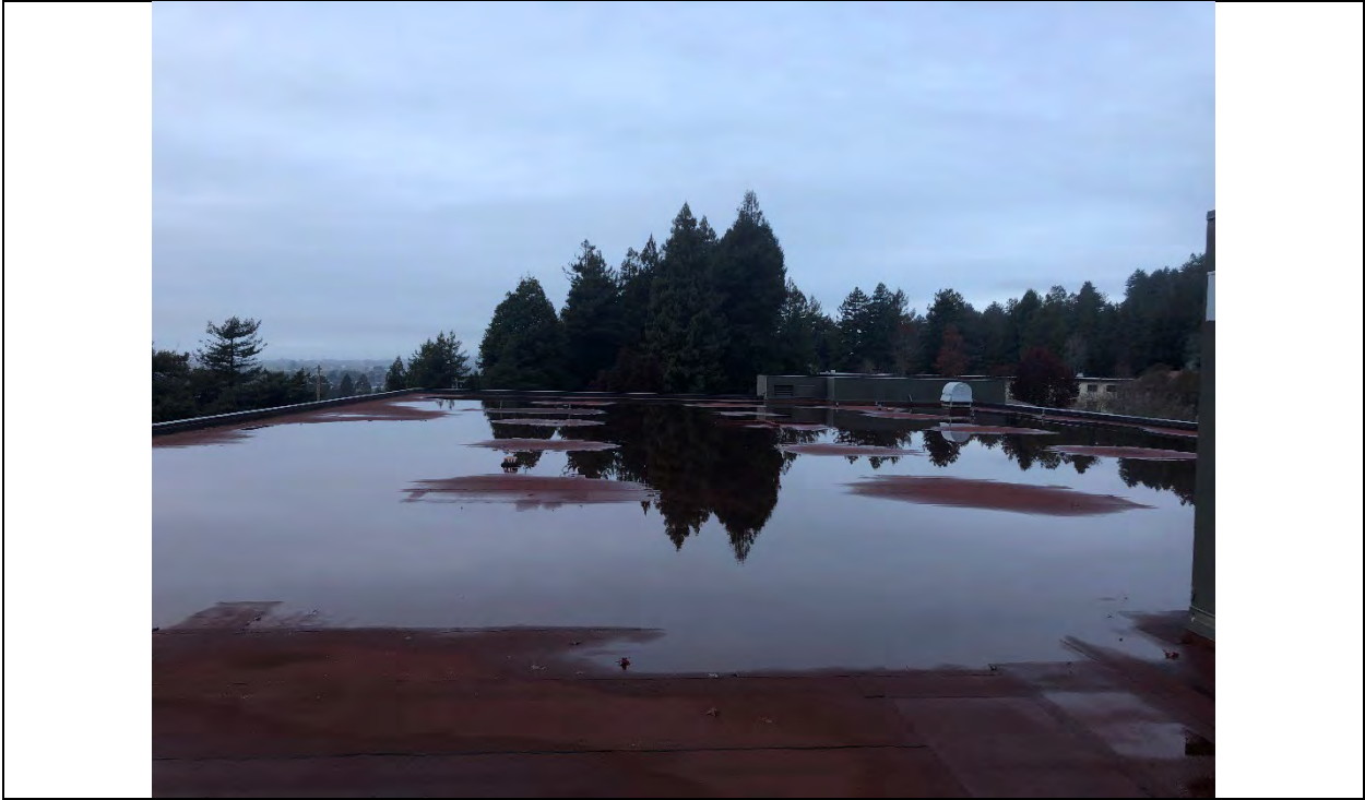
Photograph 3 – Library roof (view looking N)
