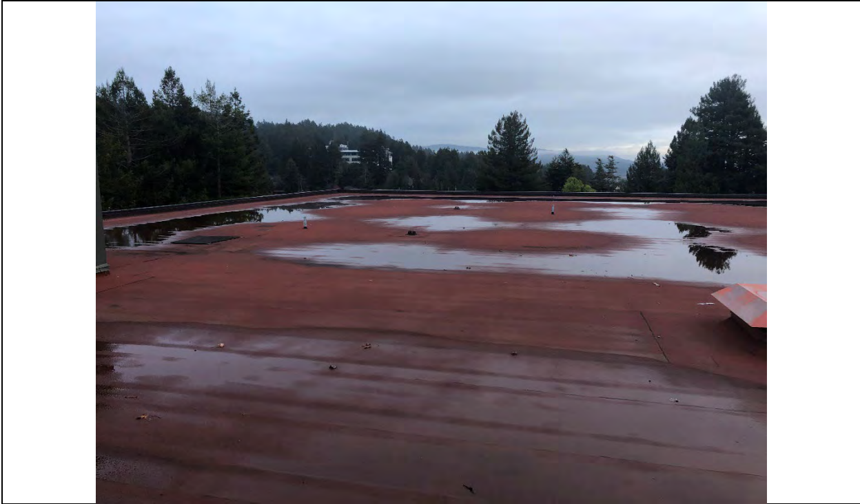
Photograph 2 – Library roof (view looking S)
