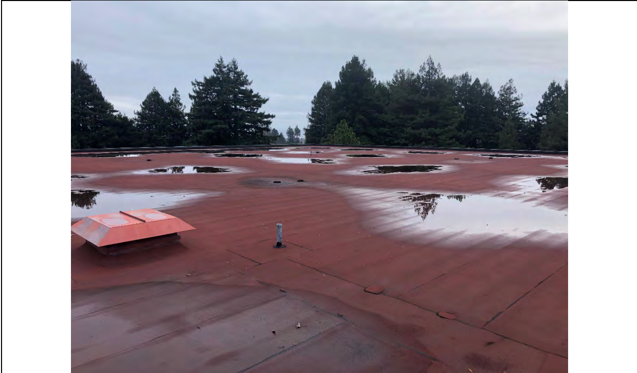
Photograph 1 – Library roof (view looking SW)
