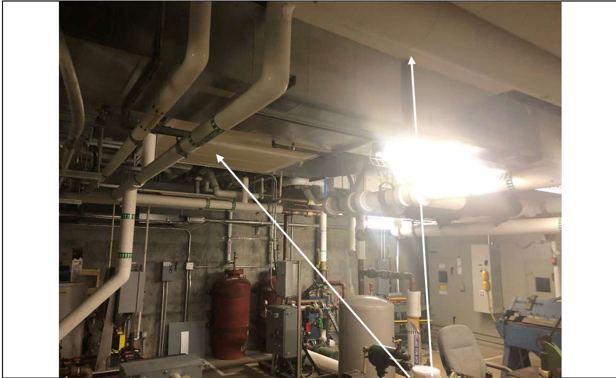
Photograph 1 – BSS Building – Room M-0A Horizontal Chase
