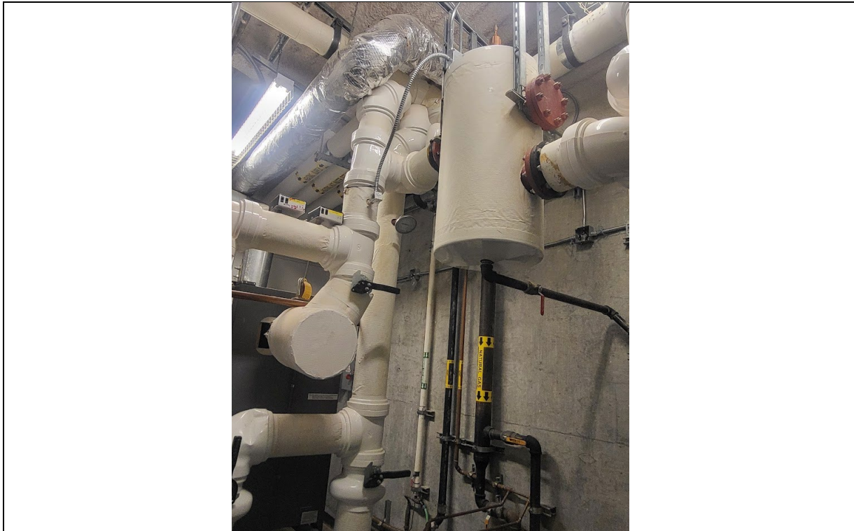
Photograph 5 – KA – Room M-3B – Fiberglass TSI (typical)
