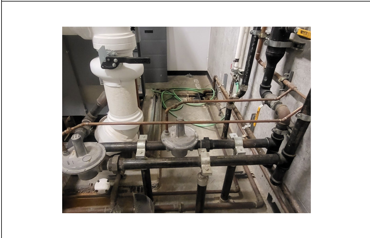
Photograph 6 – KA – Room M-3B – TSI (typical) and flange location (typical)
