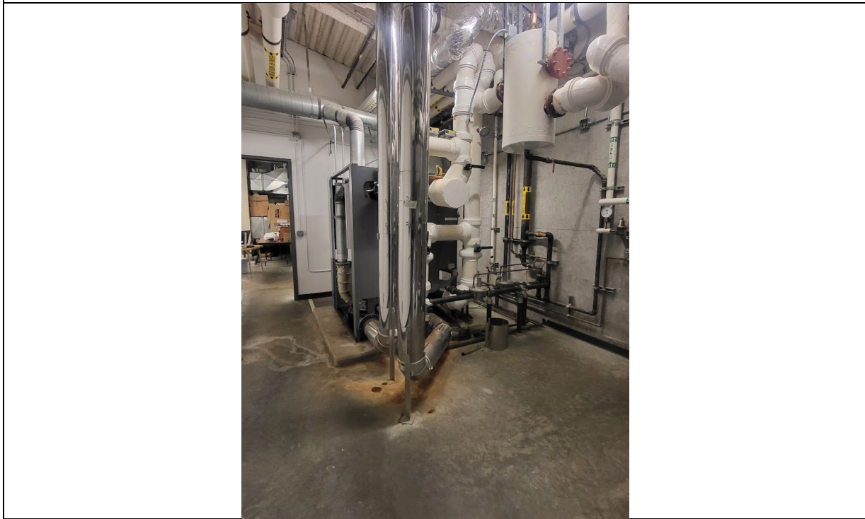
Photograph 2 – KA – Room M-3B
