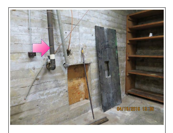
Photo 14: An asbestos-insulated pipe in Room 107, and continuing up to the second floor, and a laboratory table top stored in that room
