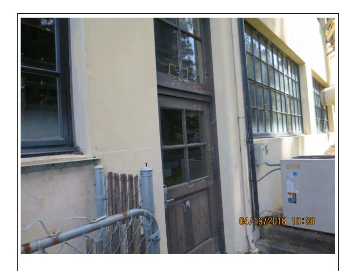
Photo 2: Lead-based paint on this wood doorway assembly
