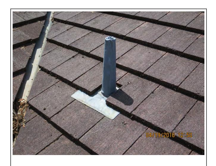
Photo 9: A typical lead vent flaqshing
