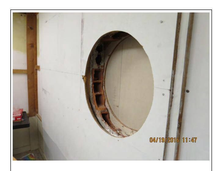
Photo 6: Except for a few newer drywall walls, the walls are made with hollow clay tile coated with plaster
