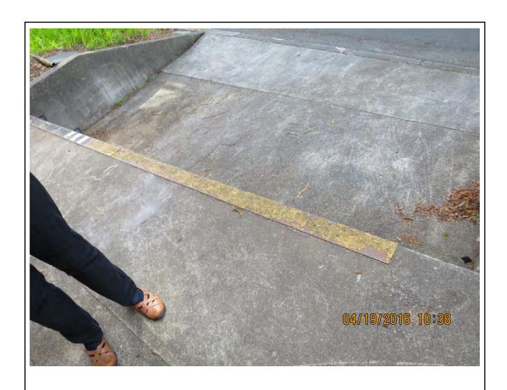
Photo 3: Lead-based paint on this metal strip at the loading dock is in poor condition
