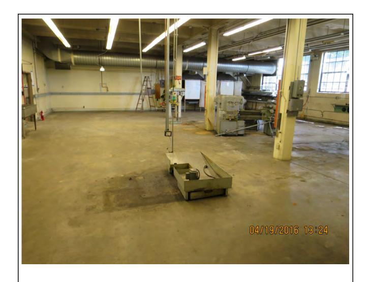
Photo 11: The former metal shop, Room 106. Note that it never had 9" x 9" vinyl floor tile as shown in a previous asbestos survey report. There are no shadow lines, nor any evidence of bead blasting
