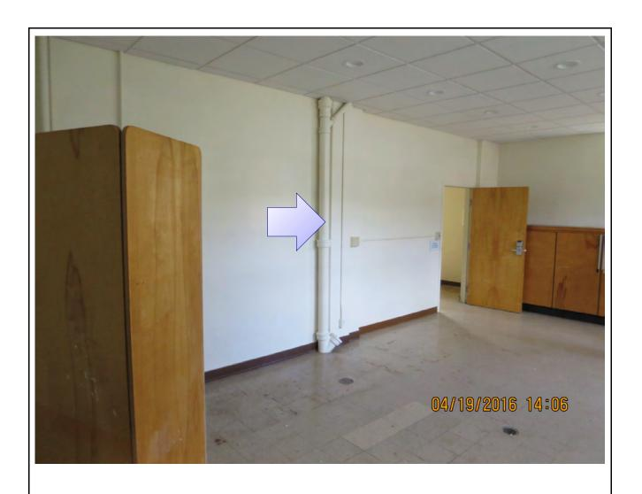
Photo 17:Room 101, and lead-based paint on the cast iron sewer pipe
