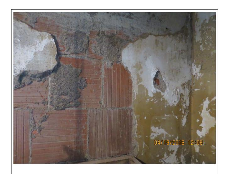
Photo 7: Another view of the hollow clay tile, hear applied on the inside of a concrete exterior wall
