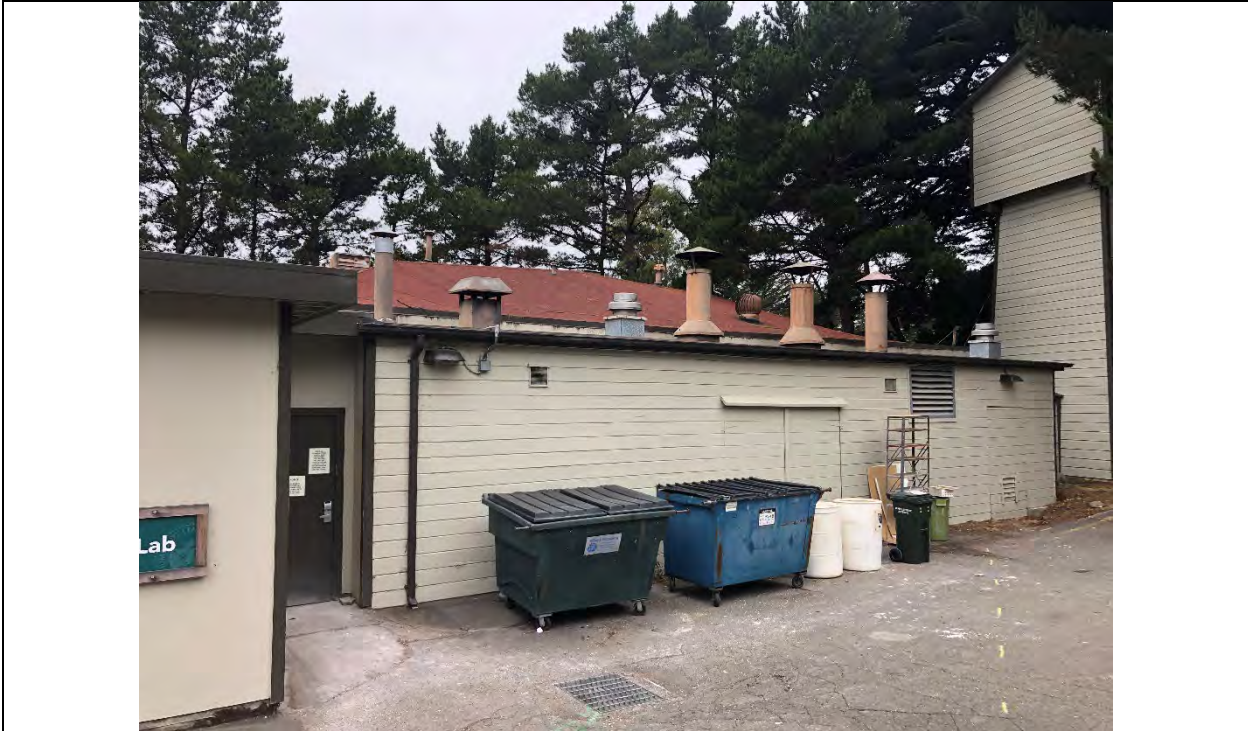
Photograph 1 – CERAM Exterior – East façade
