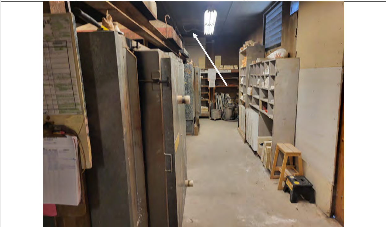
Photograph 6 – CERAM Interior – Room 108 Cementitious panel (ACM) at ceiling
