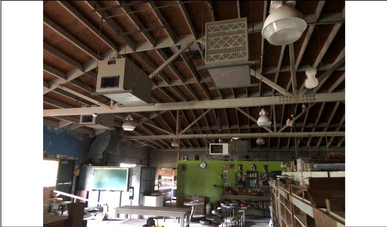
Photograph 2 – CERAM Interior – Main classroom looking east
