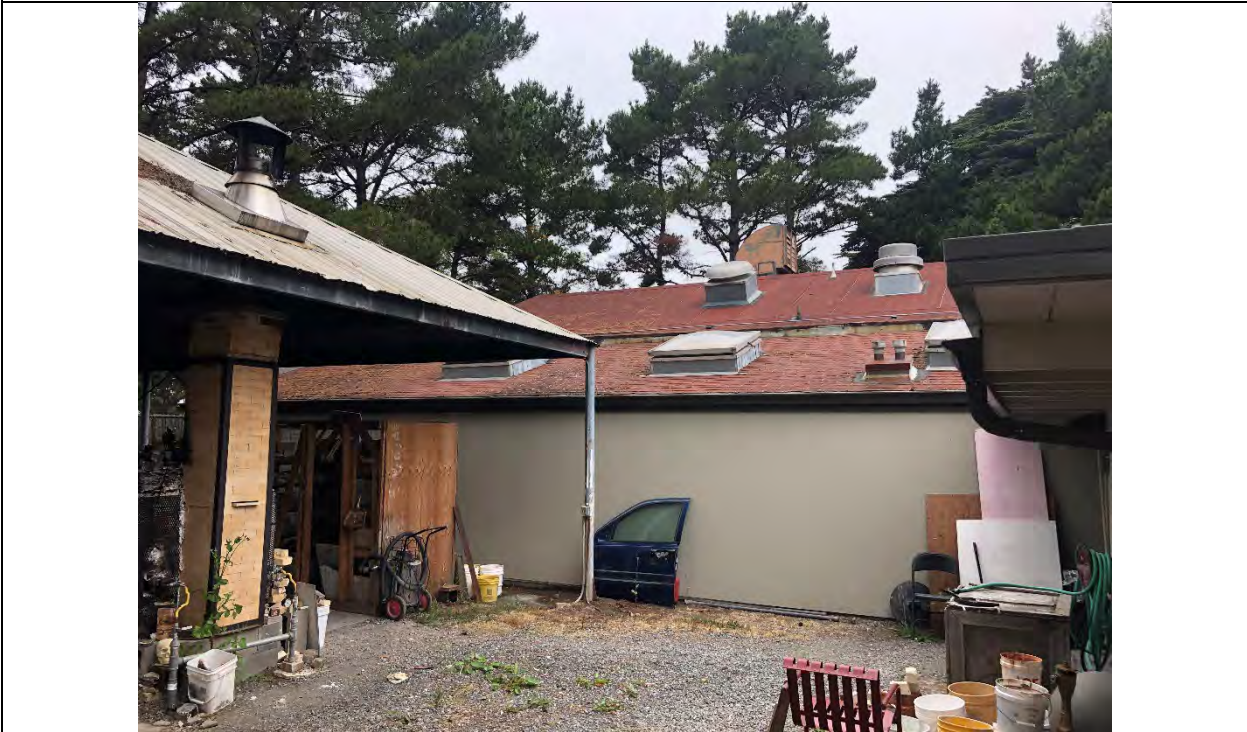
Photograph 4 – CERAM Exterior – South façade and roof
