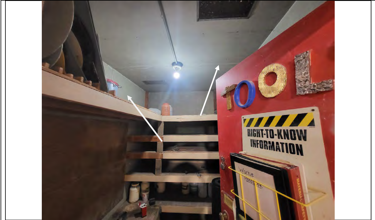
Photograph 7 – CERAM Interior – Cementitious panel (ACM) at walls and ceiling (typical)
