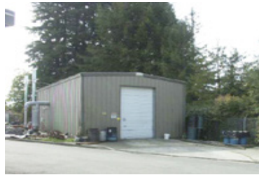
048 Hazardous Waste Handling Facility
