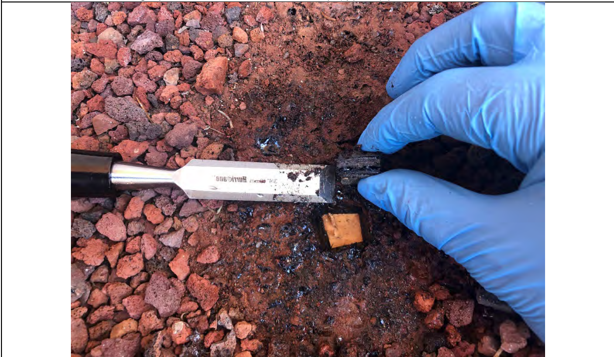
Photograph 6 – GSAC Roof – Built-up tar/ballast roof detail (typical)
