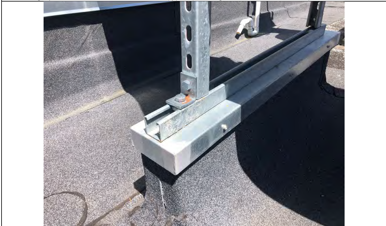
Photograph 4 – SHC Roof – HVAC support curb (typical)
