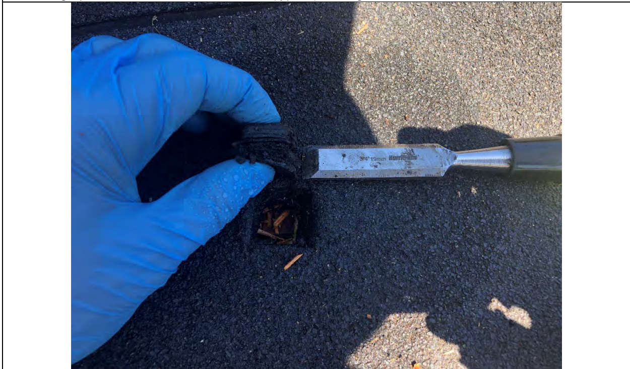
Photograph 6 – SHC Roof – Rolled roof detail (typical)
