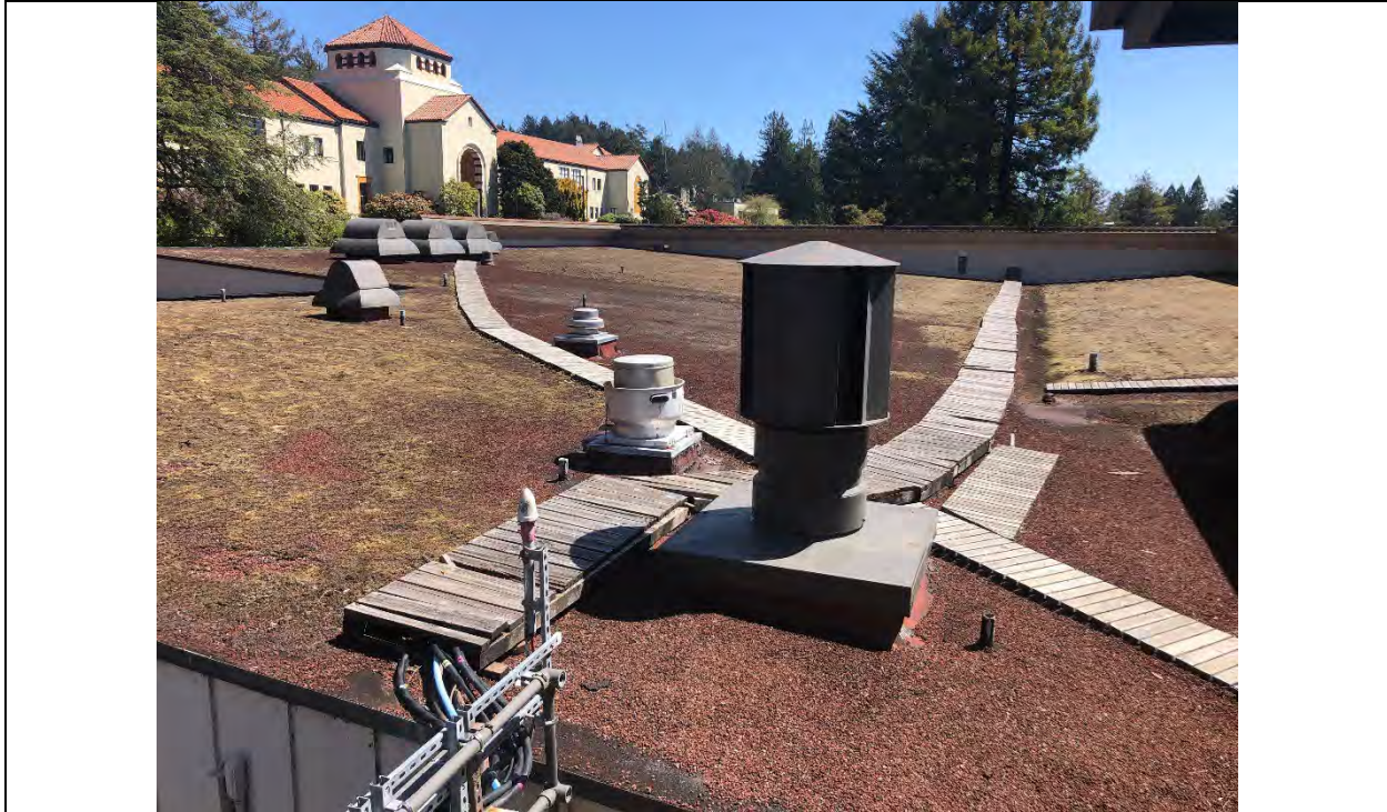
Photograph 1 – GSAC Roof – View looking southeast
