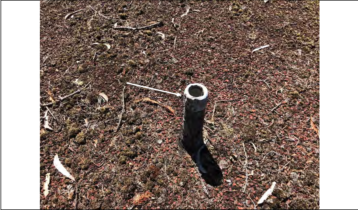
Photograph 5 – GSAC Roof – Vent cap (typical) presumed to be lead.
