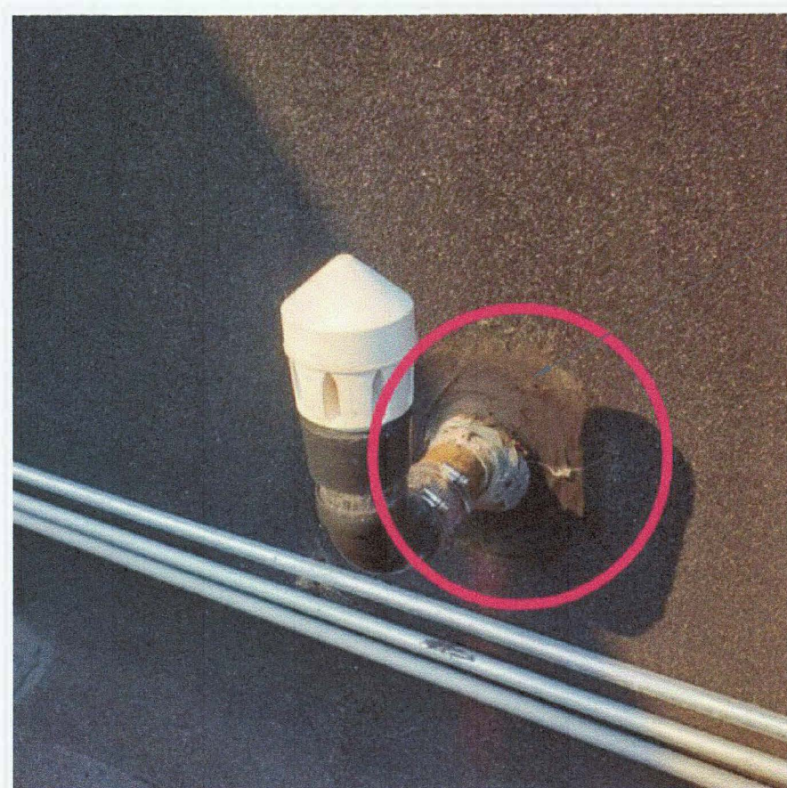
TYPICAL PENETRATION @ VERTICAL SURFACE
