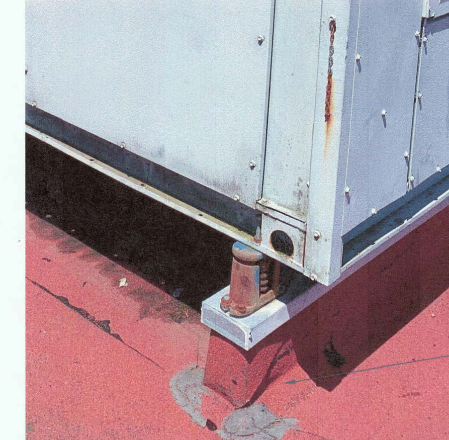
TYPICAL CURB AT MECHANICAL UNIT
