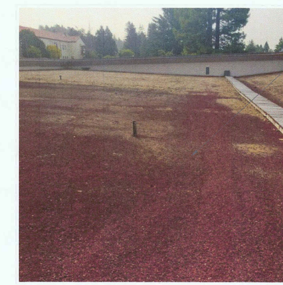
TYPICAL BALLASTED BUILT-UP ROOFING SYSTEM
