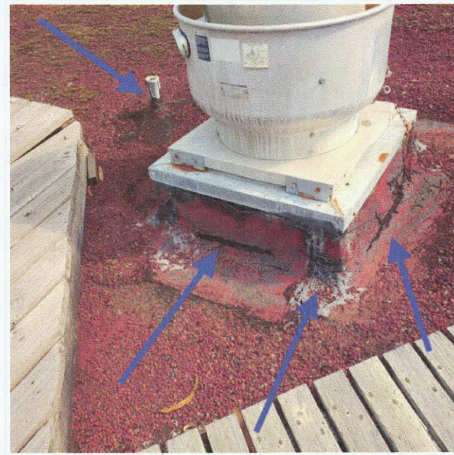
TYPICAL MECHANICAL CURB CONDITION
