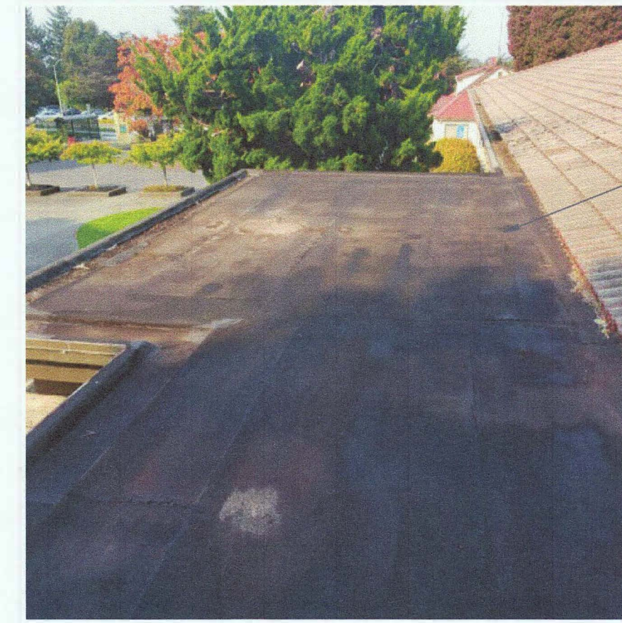
TYPICAL LOWER ROOF AREA
