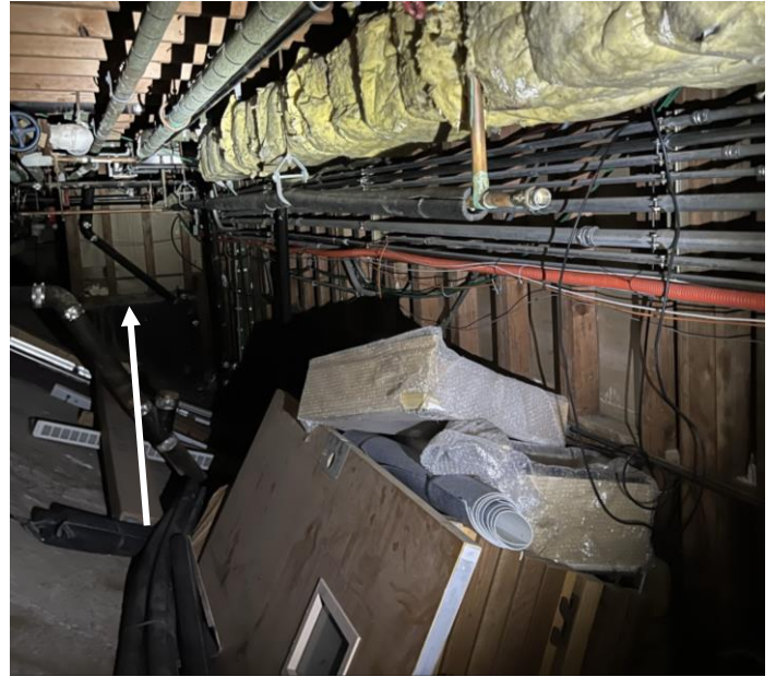
Photo 6 Maple – Basement Crawlspace – Drywall/joint compound wall and ceiling systems (indicated by arrow) associated with knock down surface texture reported to contain asbestos.
