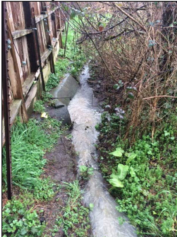
Figure 4.2B Drainage Ditch and 18-inch Concrete Pipe Inlet
