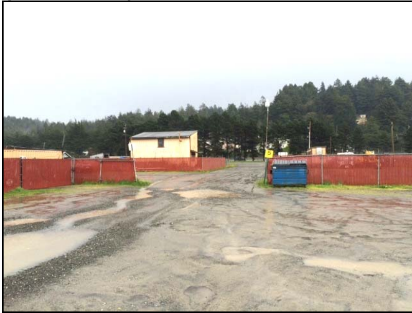
Figure 4.2C Ponding of Water on the Elevated Portion of the Site
