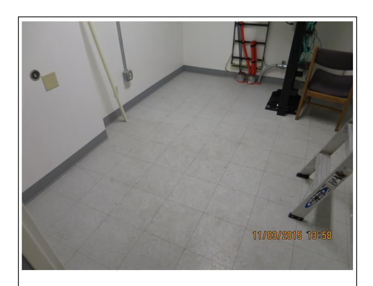
Photo 10: The new-style 12x12 vinyl floor tile in the data equipment rooms on the upper three floors
