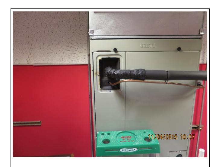
Photo 34: Black sticky tape on a refrigerant line in the former computer room in Room 111
