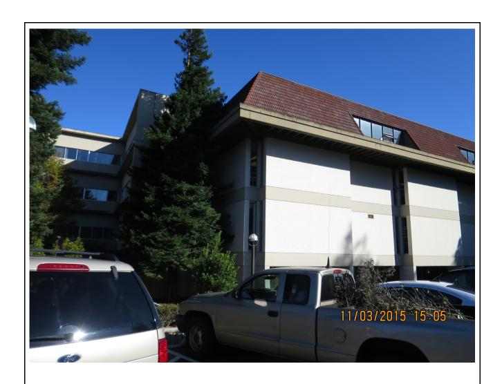
Photo 15: One view of the exterior, showing clay tile over asbestos tar paper on the sloped sections
