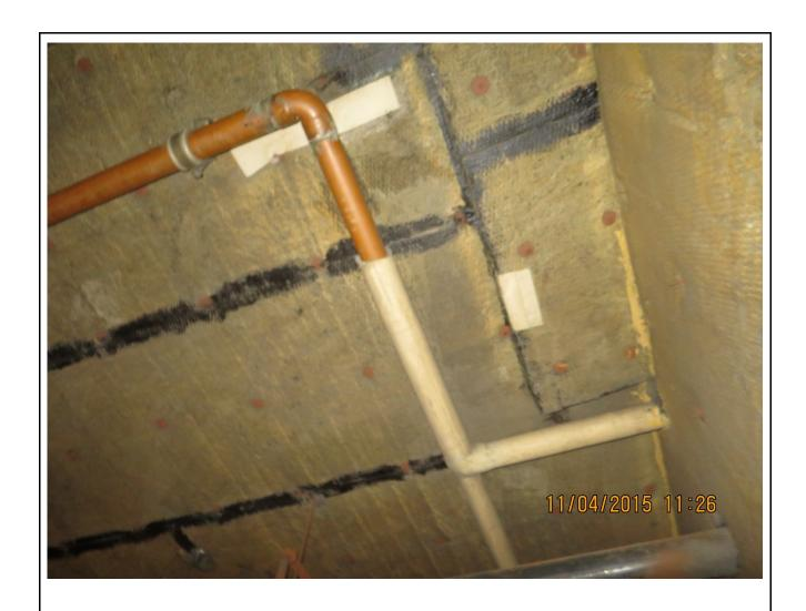
Photo 38: The exposed end of the insulation on this copper pipe labeled domestic water in the air handler fan room needs to be repaired
