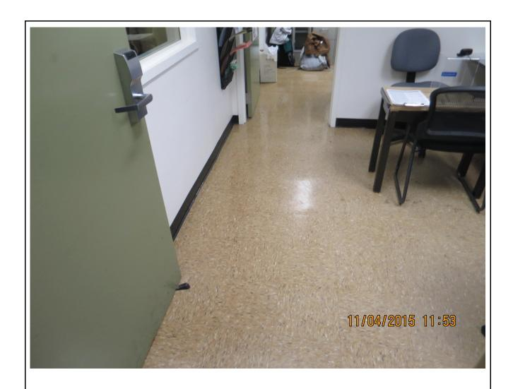
Photo 40: The typical asbestos 12x12 vinyl floor tile adhered with asbestos mastic in the basement
