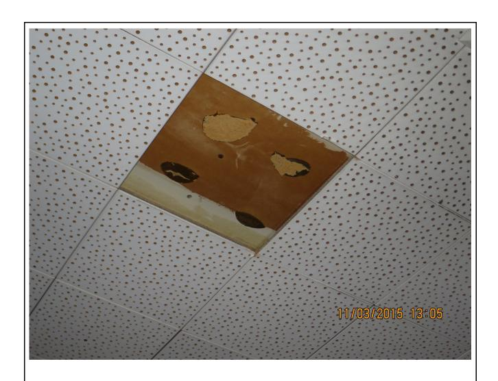
Photo 4: The 1' x 1' ceiling tile adhered with mastic, and applied to drywall with asbestos joint compound in some areas
