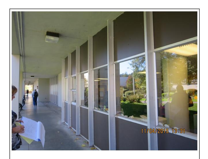
Photo 45: The brown upper and lower asbestos-cement window panels are coated with lead-based paint
