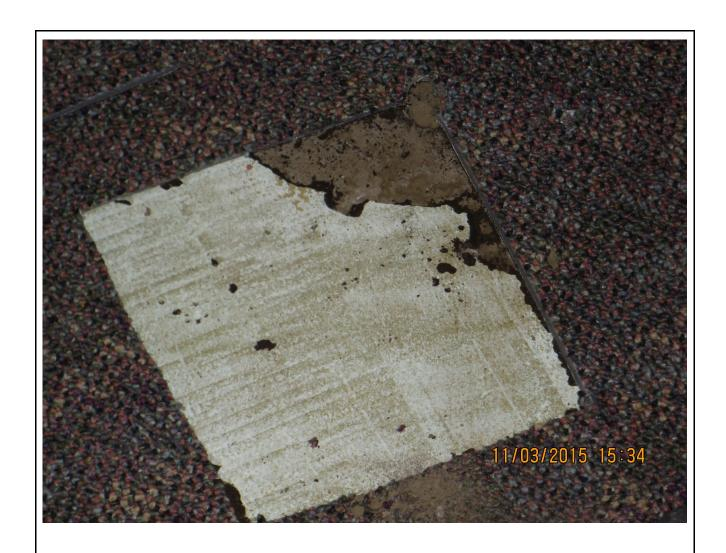
Photo 22: The coating over crumbly brown concrete in one part of the L-shaped room with the acoustic ceiling texture on the second floor
