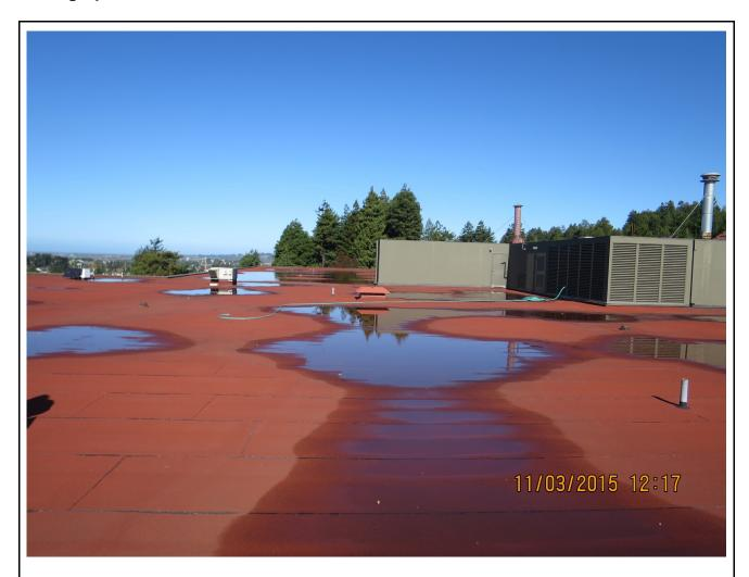
Photo 1: Severe ponding on the roof
