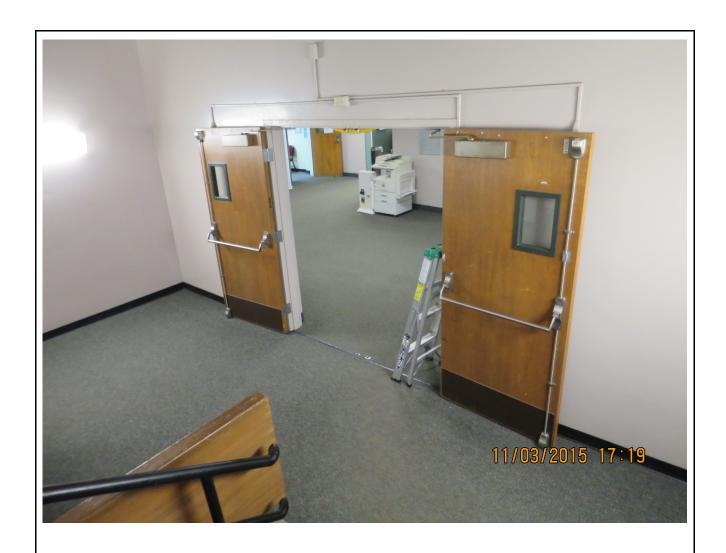
Photo 25: One of these fire door insulated with asbestos had a chip missing, exposing the insulated core
