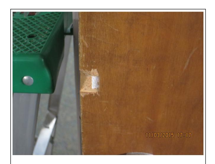
Photo 26: We applied some patching material to the exposed friable asbestos fire door insulation at the location where the door was chipped on the first floor
