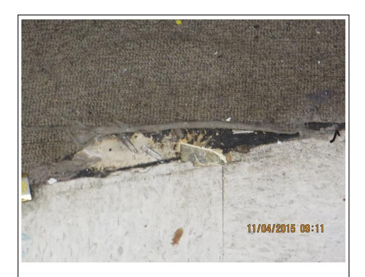
Photo 29: The two layers of 12x12 vinyl floor tile behind the main counter on the first floor, bottom layer is adhered with asbestos mastic
