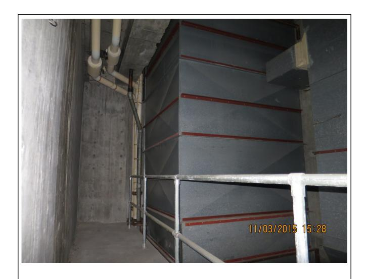
Photo 21: Pipes with fiberglass insulation and canvas duct seam tape in the duct chase
