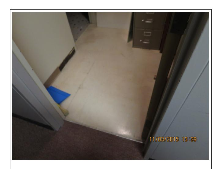
Photo 9: The old 9" x9" vinyl floor tile adhered with asbestos mastic on the 3<sup>rd</sup> Floor is exposed in these two former restroom (now abandoned) entry areas
