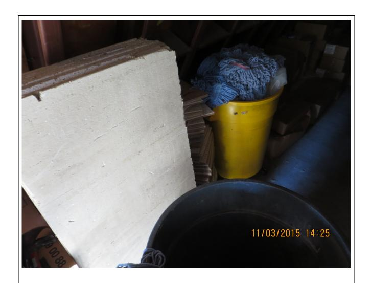
Photo 14: Spare new non-suspect type 2' x 4' suspended ceiling panels and old 1' x 1" ceiling tile which have been removed and stored
