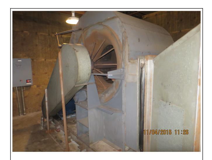
Photo 37: The large fan and the non-suspect fiberglass and "rubber" flexible duct connector in the air handler rooms next to the boiler room in the basement
