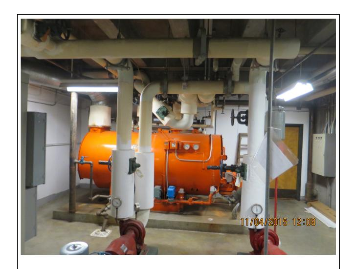
Photo 41: The newer orange boiler is coated with lead-based paint, but the piping is insulated with fiberglass
