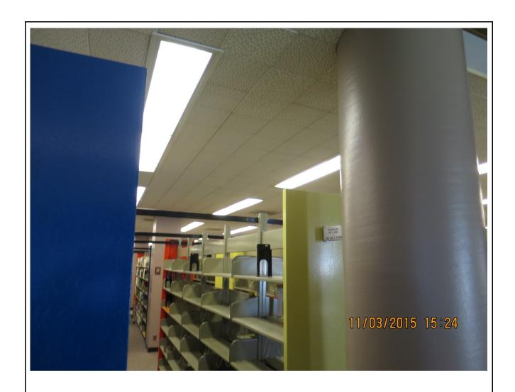
Photo 19: Wood fiber ceiling tile on the north end of the second floor
