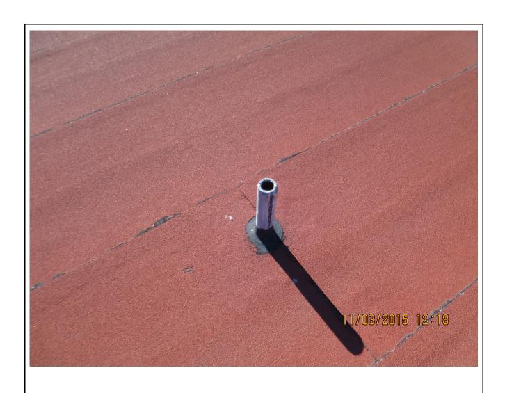
Photo 2: Typical lead flashing on a vent
